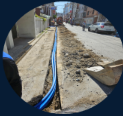
Placing Microduct
